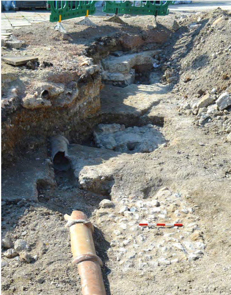
Fig. 52 Early pier base 146 after machine reduction, looking west. Piers 152 and 101/142 in background. Scale, 50cm
