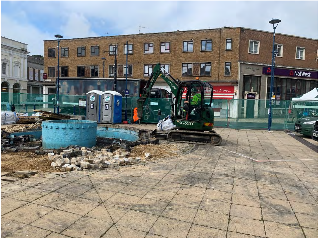
Fig. 36 Machine removal of the 1980s fountain, looking west
