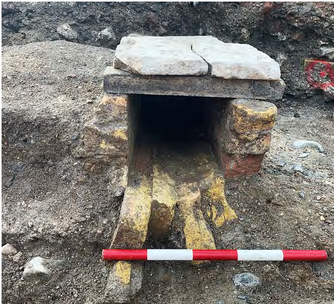
Fig. 56 Nineteenth century brick culvert 108 in Area 1, looking south; possible overflow to the town pump
