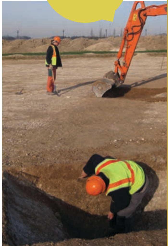
Topsoil stripping © CG62
